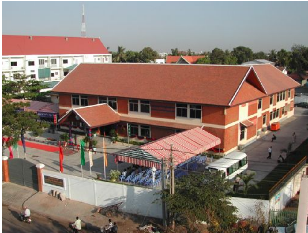
Inland Fisheries Research and Development Institute (IFReDI) building located in Phnom Penh, Cambodia.
